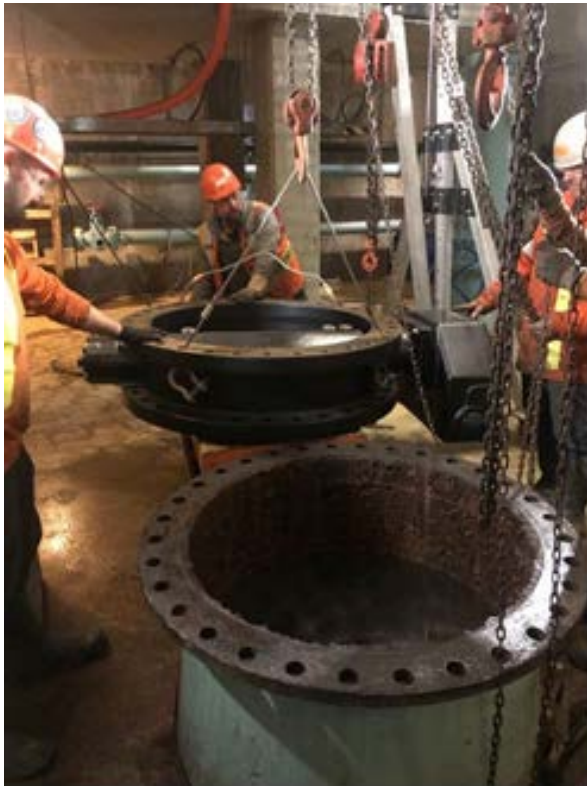
Figures 6a and 6b: Replacement of the 36" suction isolation valve on HLP #3.
