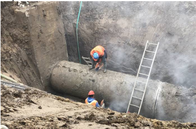
Figure 7b: Cutting into the pipe to perform the repair.
