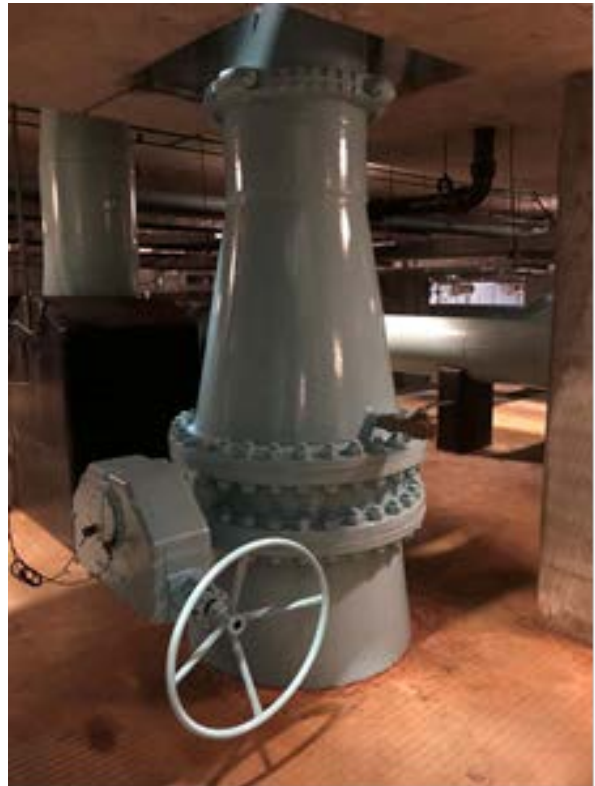
Figures 6a and 6b: Replacement of the 36" suction isolation valve on HLP #3.
