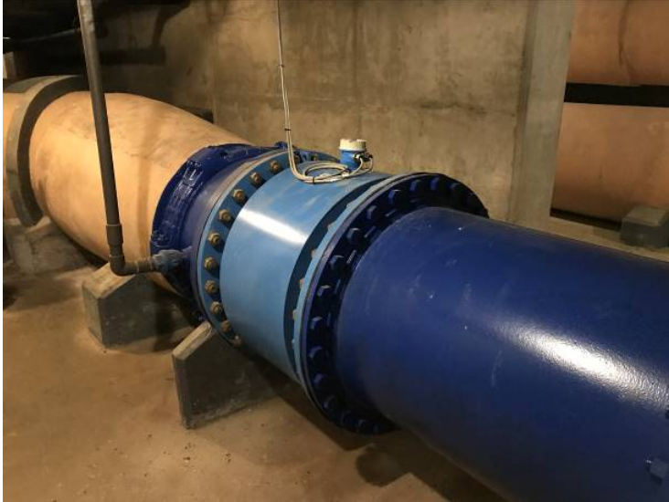
Figure 5: New raw water flow meter, north side.
